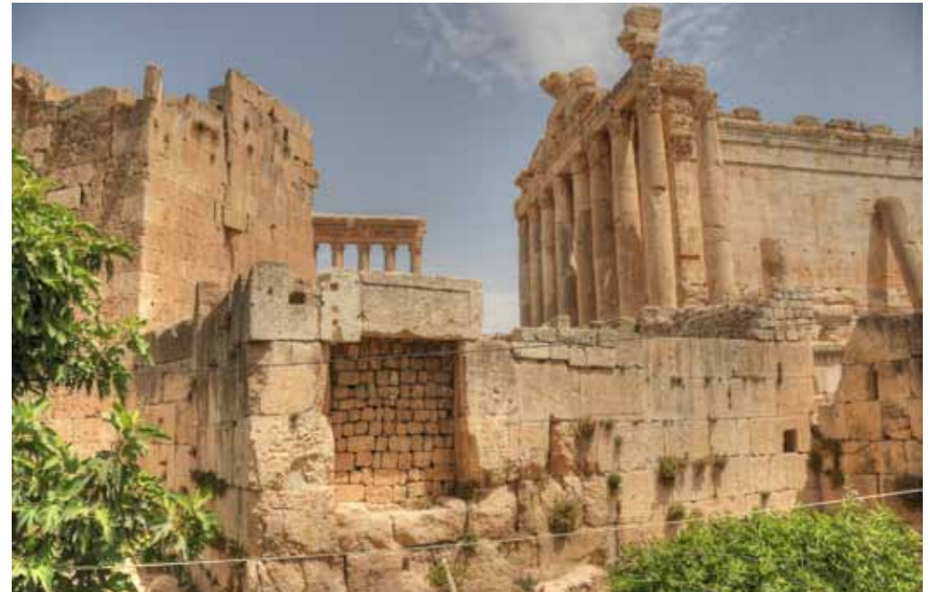
Figure 12: western wall, foundations and Bacchus temple, author
